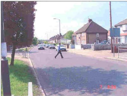
Manor Farm Road - Inadequate crossing facilities
